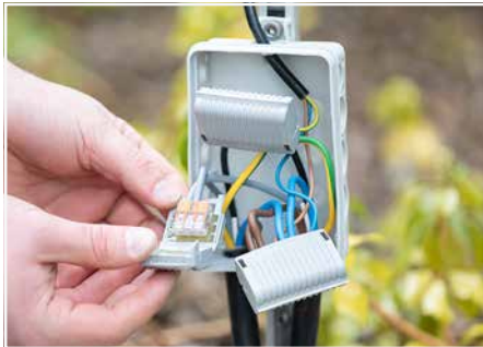
Connecting a bollard light
