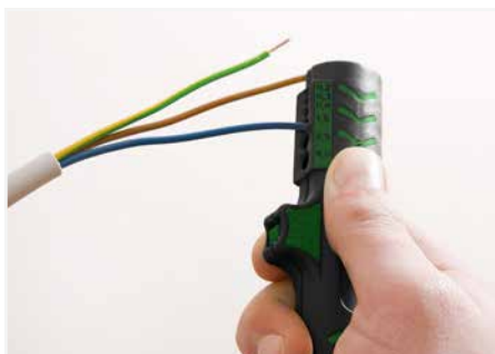
Stripping a conductor insulation.
