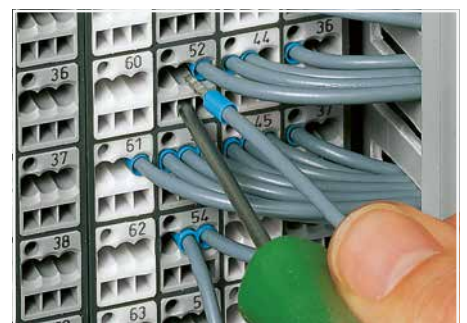
Terminating ferruled conductors via operating tool.
