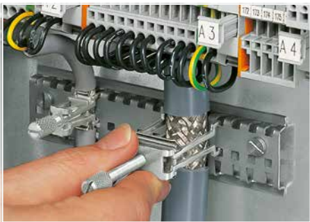
Securing an additional shield clamping saddle.
